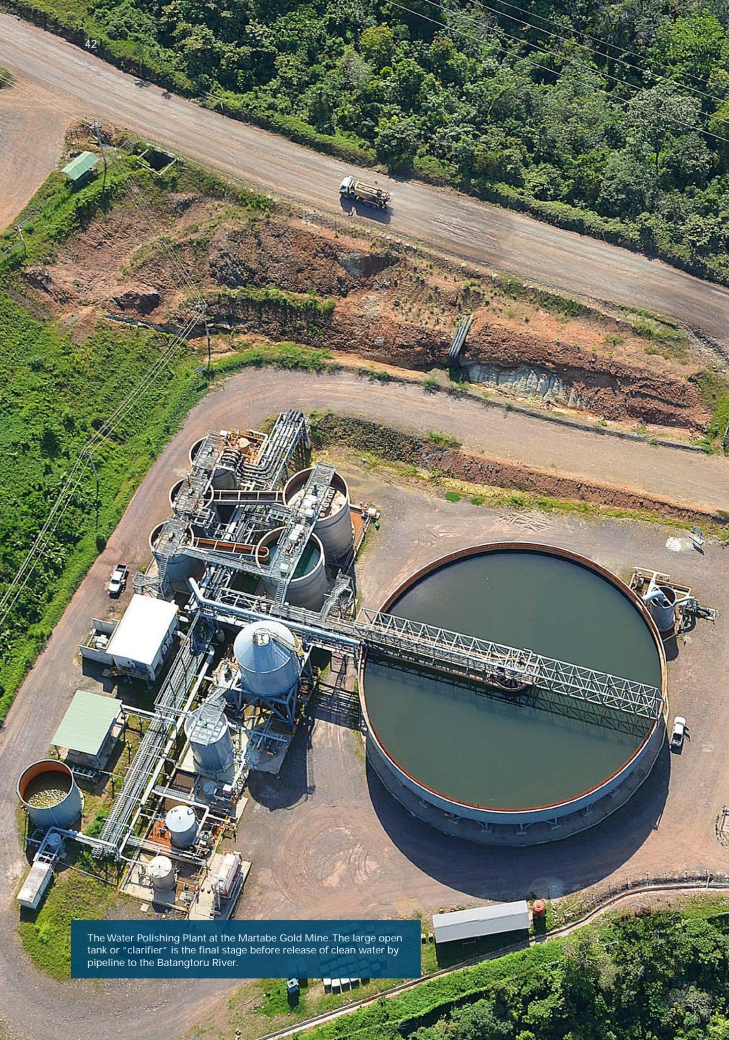
The Water Polishing Plant at the Martabe Gold Mine. The large open tank or "clarifier" is the final stage before release of clean water by pipeline to the Batangtoru River.
