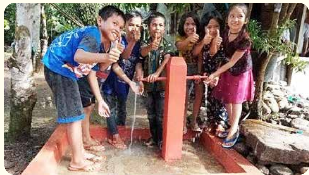
5 November 2020 PTAR builds clean water facilities in the Batuhoring Village, Batangtoru.
