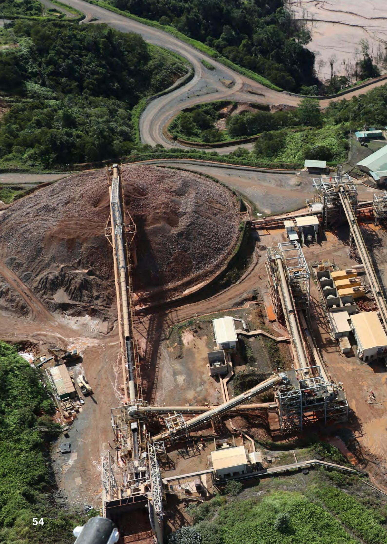
View of the Martabe Gold Mine process plant (ROM stockpile on the left, grinding mills in the centre, and leach tanks on the right).
