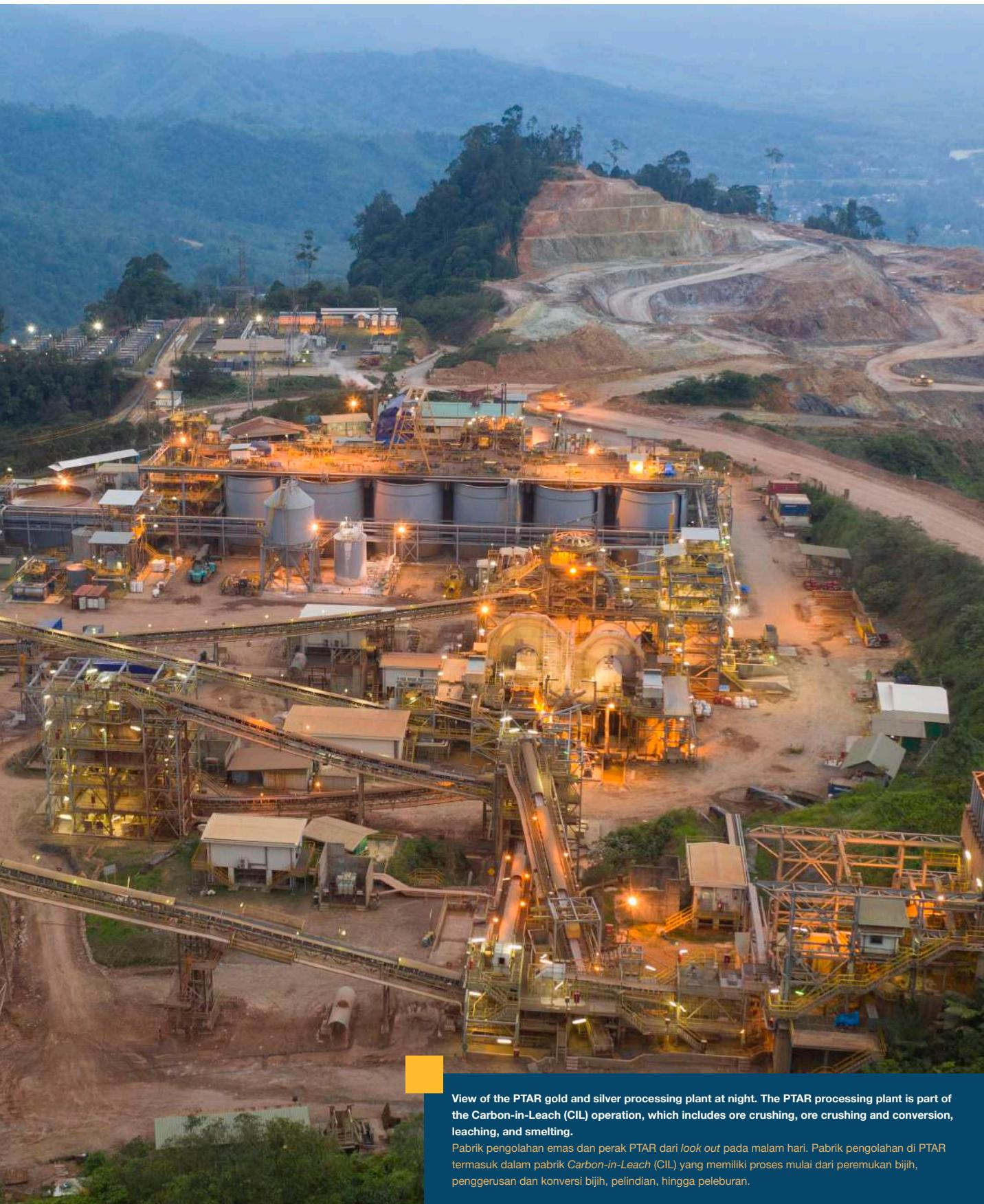
View of the PTAR gold and silver processing plant at night. The PTAR processing plant is part of the Carbon-in-Leach (CIL) operation, which includes ore crushing, ore crushing and conversion, leaching, and smelting.
