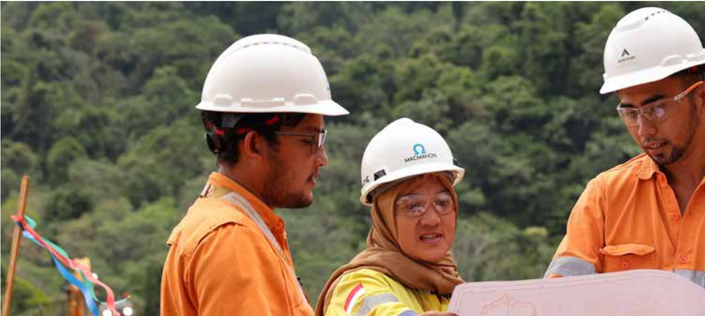
The Martabe Project Development Team of PT Agincourt Resources (PTAR) and its work partners monitor the progress of the Tailings Management Facility (TMF) construction. The TMF is one of the tailings storage facilities prepared by PTAR using dewatering and filtration technology.
